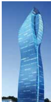
TUNED MASS DAMPERS
